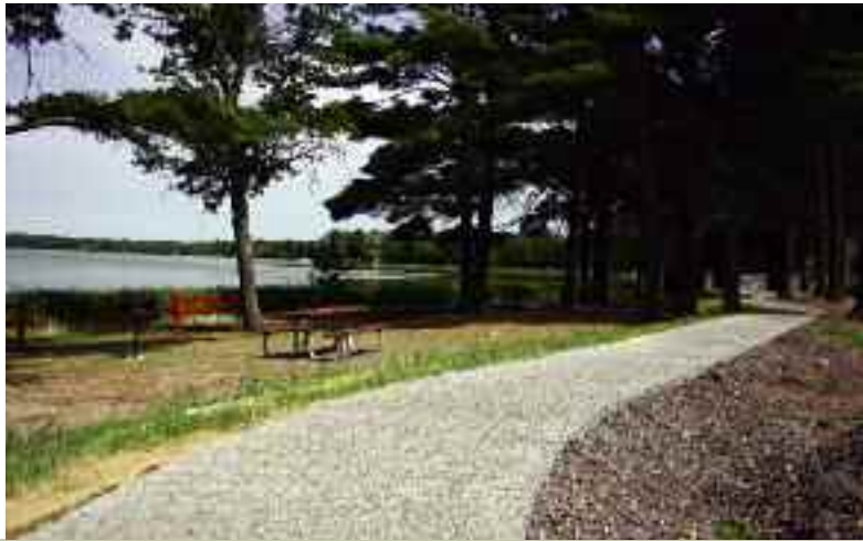
Porous concrete sidewalk at the Clam Narrows boat landing in Burnett County.
